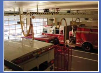
Photos of the Centereach Fire Department Station 3 with newly added Bunker Gear Rooms and Truck Bay Exhaust System
