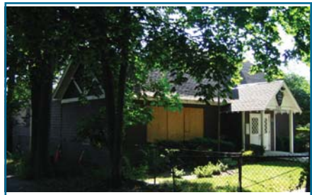
Original Building with Fire Damage Before Renovations
