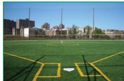
Completed recreation center ball field
