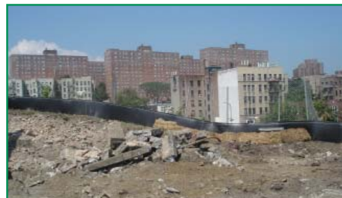
West Bronx recreation center ball field under construction
