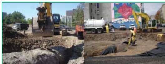
West Bronx underground oil storage tank removal
