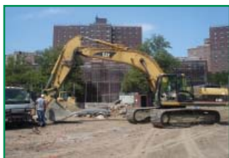
PS-29 ball field construction
