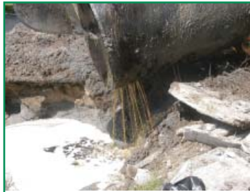
Underground Oil tank removal after evidence of leaking
