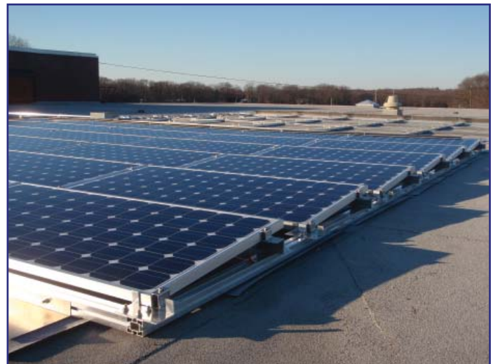
Smithtown School District Solar Panel Installation Project
