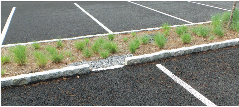
pervious paving with bioretention islands
