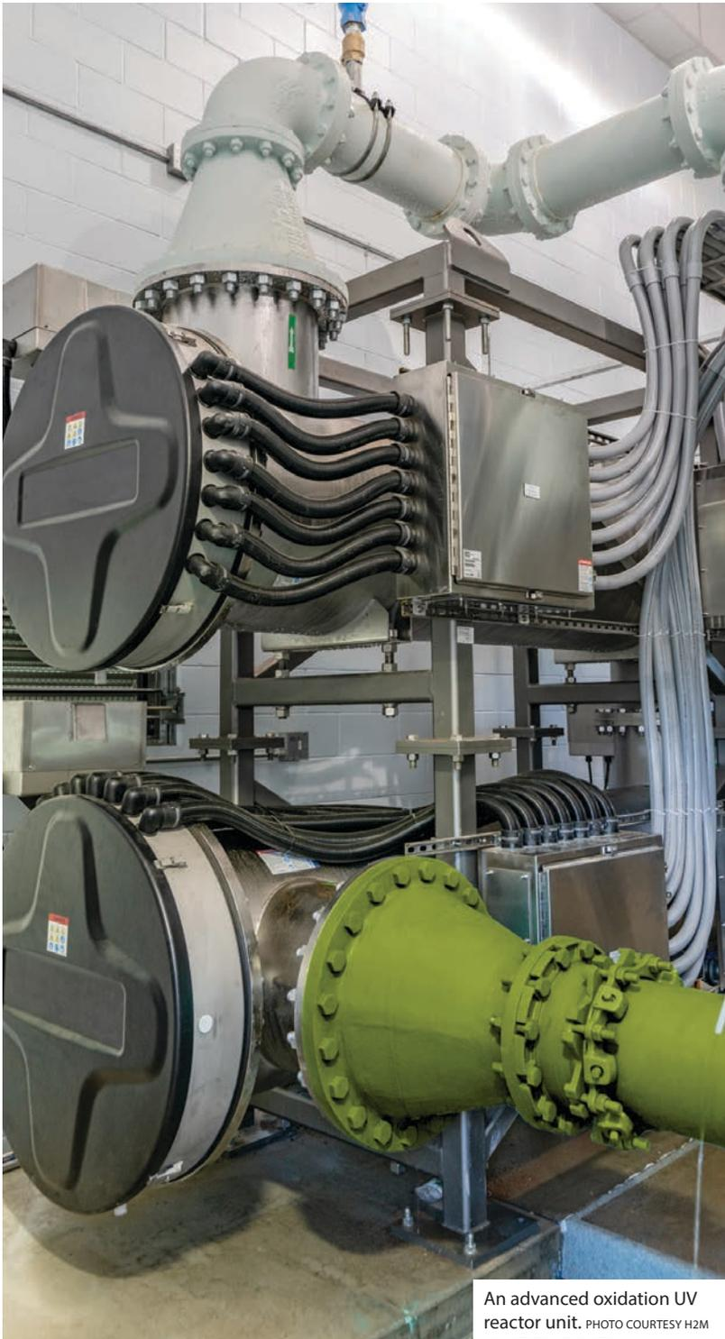
An advanced oxidation UV reactor unit. PHOTO COURTESY H2M ARCHITECTS + ENGINEERS
